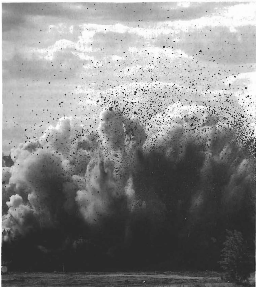
Figure 19.1 Flyrock during blasting.
